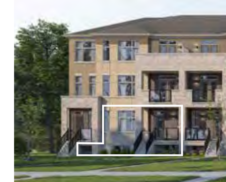
FRONT, Interior Unit
